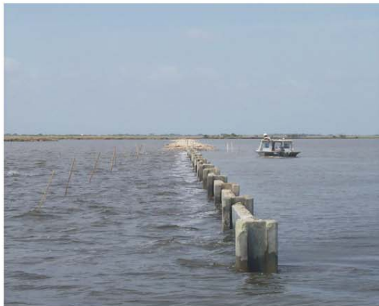
Concrete "H" pile/panel structures, similar to this one, will be installed at locations within the project area where shoreline erosion is critical. Soils with high amounts of organic material, which have poor strength, necessitated the use of a structure such as this.
